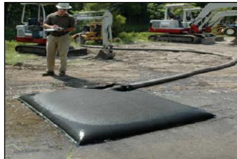
Plate 4.2 Silt bag under inspection
